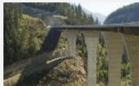
Koking Horse Canyon Tunnel, Canada
